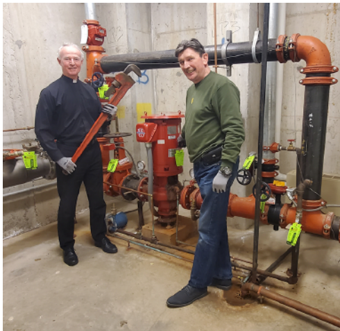
Replace fire pumps in Church and Ed Center
